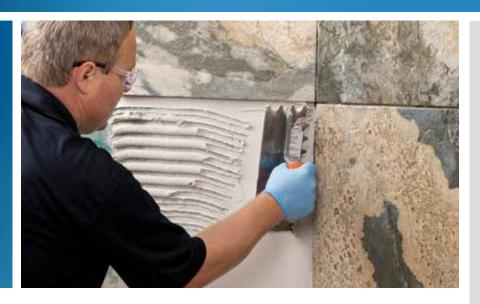
The ISO 13007 standards express product classifications alphanumerically, using simple letters and numbers. Letters describe the chemical nature of the adhesive (such as cement-based, mastic, epoxy or urethane) along with special characteristics (such as fast-setting, slip-resistant or deformable). Numbers indicate whether the product performance is "normal" (such as normal in bond strength, for light to medium traffic use) or "improved" (such as higher in bond strength, for high traffic use).
