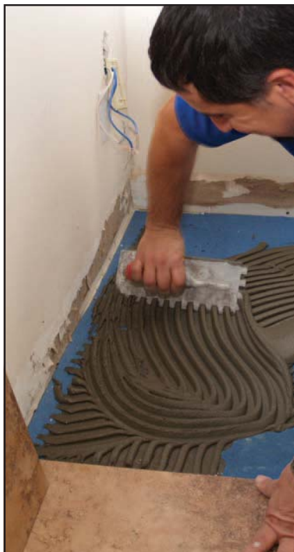
Granirapid flexible mortar system was used to install 20,000 sq. ft. (1,858 m 2 ) of porcelain tile on the building's upper level.
