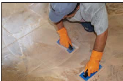
Kerapoxy chemical and stain-resistant grout was used to grout 35,000 sq. ft. (3,252 m 2 ) of porcelain tile throughout the building.
