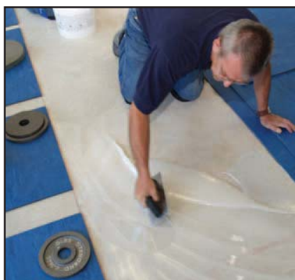
Ultrabond G21 polyurethane-based adhesive was used to install large-format rubber tile in MAPEI's employee gym.
