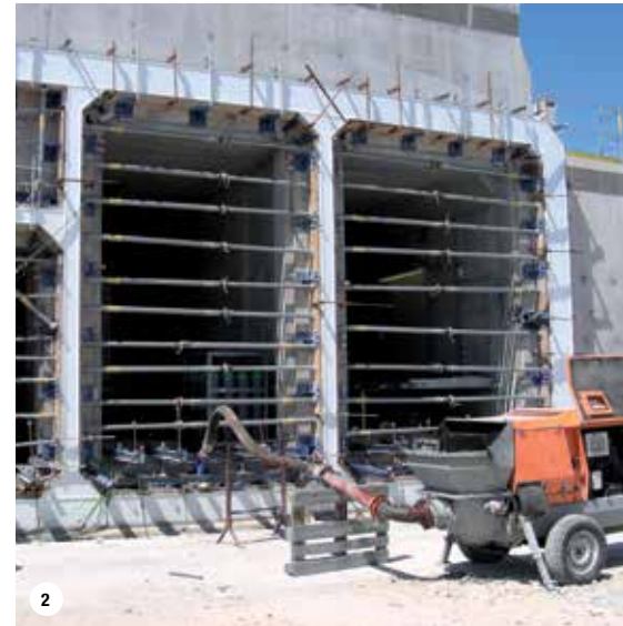
1. Reinforced concrete caissons used in the MOSE project during their manufacture. The joint housings for the caissons were connected together with a jointing system made up with Mapefill MF 610 . 2. Preparing and positioning formwork on the caissons before pumping Mapefill MF 610 .
