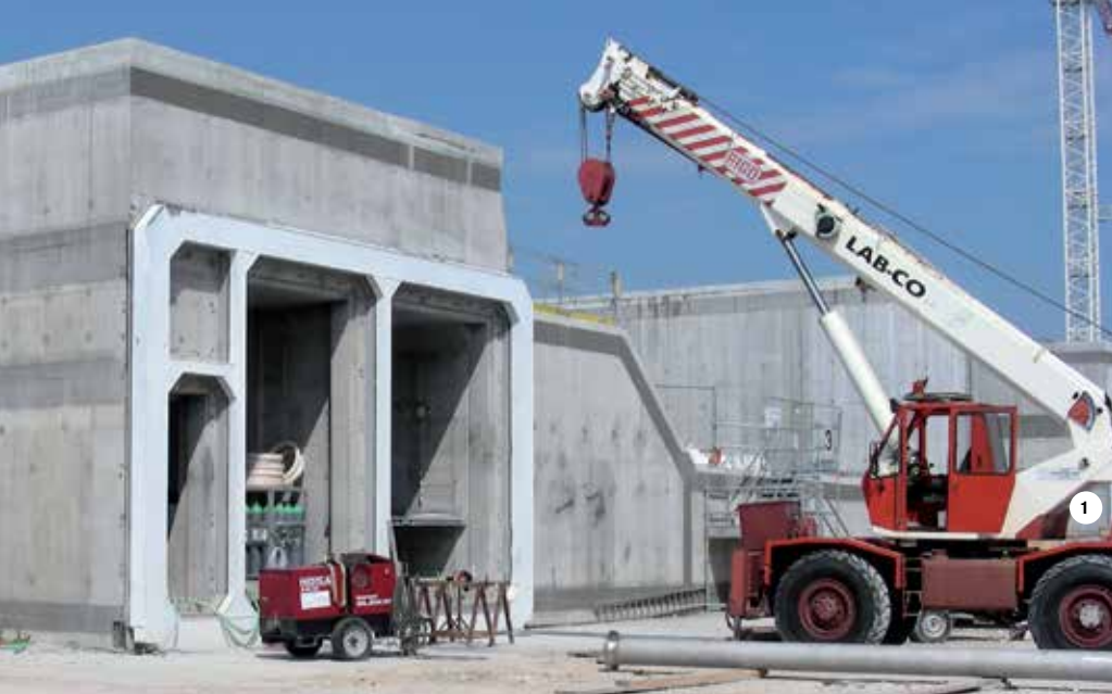
1. Reinforced concrete caissons used in the MOSE project during their manufacture. The joint housings for the caissons were connected together with a jointing system made up with Mapefill MF 610 . 2. Preparing and positioning formwork on the caissons before pumping Mapefill MF 610 .
