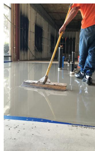
MAPEI's ESPS is based on robust, epoxy moisture-barrier solutions combined with specifically engineered cement-based leveling compounds that have been designed to withstand extremes in temperature, liquid or freezing water exposure, and the rigors of construction traffic.
