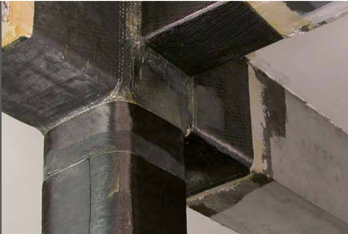
Fabrics easily adaptable to the shape of structural members
