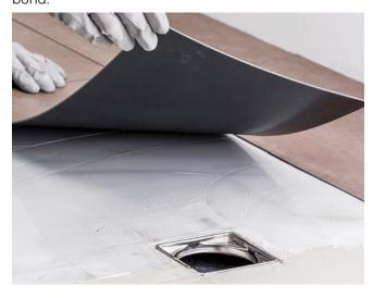
Existing floor and wall coverings made of ceramic, porcelain, or natural stone tiles must be well bonded to the substrate and free from substances that could affect the adhesion of the membrane, such as grease, oil, paints and wax. To remove such substances, use suitable cleaning products and/or abrade the surface.
