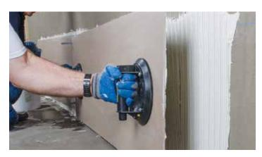
When dealing with tiles that may be as large as 5 by 10 ft. (1,52 by 3,05 m), the installer can appreciate how extra time significantly enhances the ease of application.
