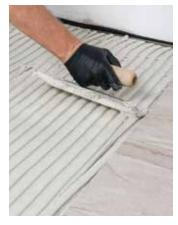
Spread only as much material as can be covered with tiles before the mortar dries or loses tackiness to the touch
