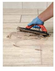
Remove excess grout from the tile surface by holding the rubber float at a 90-degree angle (perpendicular to the tile surface) while moving it across the tile in a diagonal direction.
