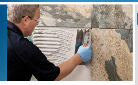
The standards express product classifications alphanumerically, using simple letters and numbers. Letters describe the chemical nature of the adhesive (such as cement-based, mastic, epoxy or urethane) along with special characteristics (such as fastsetting, slip-resistant or deformable). Numbers indicate whether the product performance is "normal" (such as normal bond strength, for light to medium traffic use, etc.) or "improved" (such as higher bond strength, for high traffic use, etc.).
