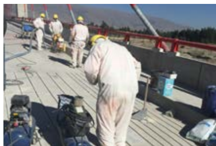
Aplicação de barras de carbono pultrudidas. Application of pultruded carbon fibre rods.
