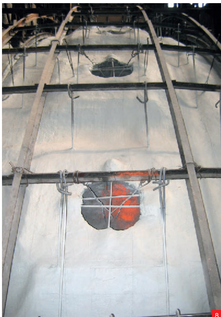
Photo 5. Preparation work before laying MapeWrap C UNI AX.
