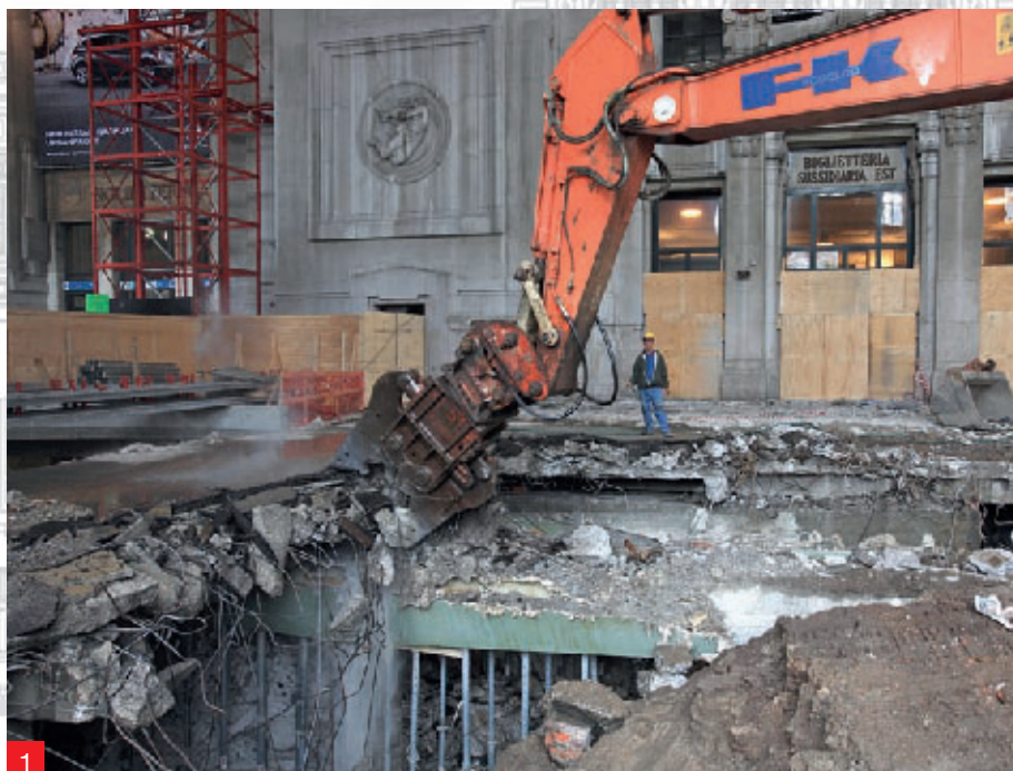
Photo 1. Demolition of the old floor.
