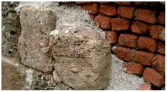
A problem often encountered in buildings, both historical ones and those built more recently, is deterioration of the masonry and construction elements. These structures require the right operations; sometimes they may need consolidation work, other times to be renovated or they are in need of conservative restoration.
