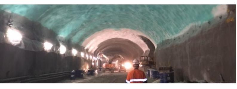
**Lamposilex** and **Planiseal 88** repair products were used before spraying the membrane to plug and patch any areas with water in-flows.
