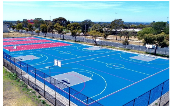
After Mapecoat TNS Comfort System
