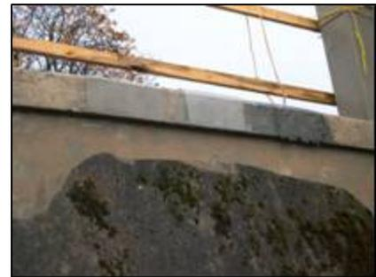
The original coping atop the seawall had become too eroded and damaged from exposure to the harsh sea air for the renovators to apply the *Planitop 12* directly to the wall. Before beginning the
