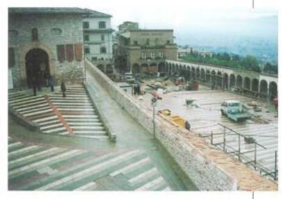
Marble sheets of various dimensions but uniform thickness - 10 cm - were laid in an end-to end configuration, with joints of 1.5 cm. Planners aimed to make the surface suitable for pedestrian traffic.
