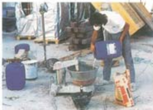
Mixing Kerabond and Isolastic
