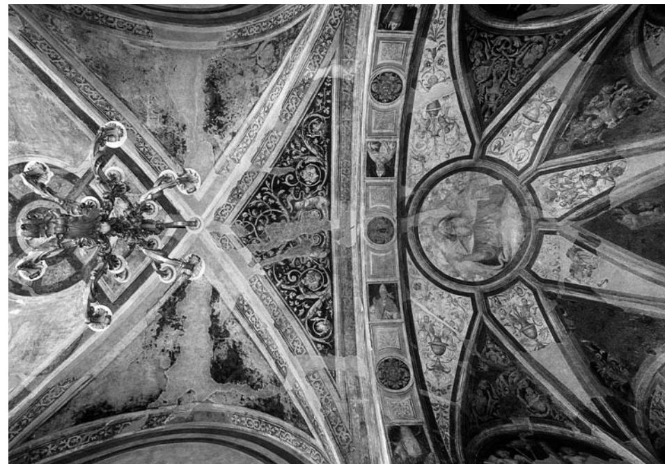
Detail of the hall and apse vault after completing repairs.
