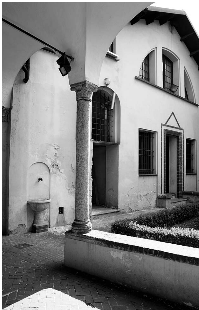
Main façade of the Oratorio della Passione before repairs.
