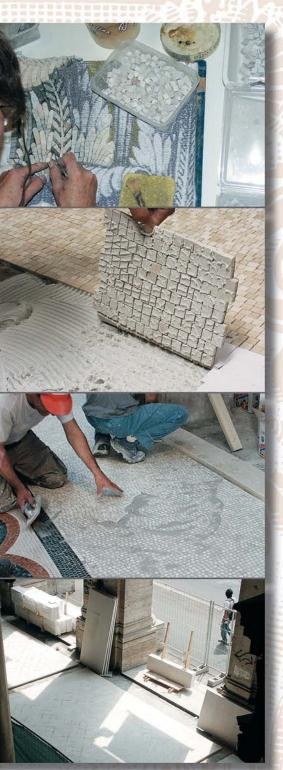
rative mosaic.TOPCEM\* mixed with gravel varying in grain size from 0-8 mm for thickness ranging between approximately 4-6 cm was used for making the screeds inside the areas designed for holding shops.
