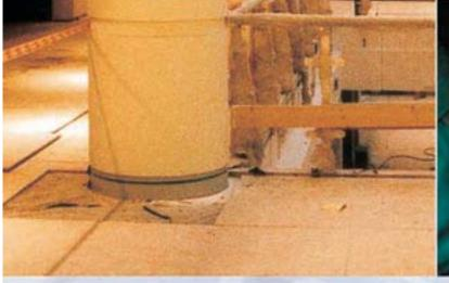
For installing ceramic tiles on the floors, the investor initially opted for self-filling tile adhesives with semi-liquid consistency.
