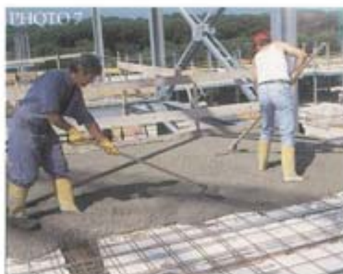
Photo 7 The surface of the pour was smoothed manually.
