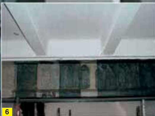
Photo 7. Close-up of the shear strengthening.
