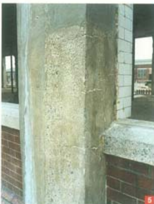
Photo 5. The structure of this column was reinstated with MAPEGROUT after repairing the steel.
