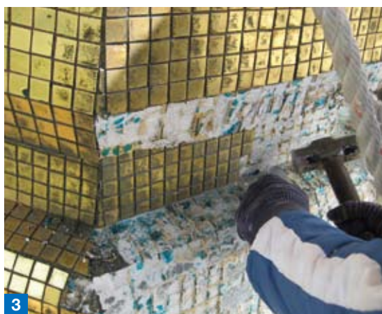
Photo 4. Once old mosaics were removed, the original surface came to the light.
