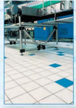
\*Mapei Products: the products referred to in this article belong to the "Products for Ceramic Tiles and Stone Materials" range. The technical data sheets are available on the "Mapei Global Infonet" CD/DVD and from the web site: www.mapei.com. Mapei adhesives and grouts conform to EN 12004 and EN 13888 standards. Adesilex P22 Plus (D1TE): ready-touse paste adhesive for laying tiles on internal walls. N.B. This product is only
