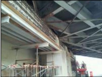
Because of its elaborate design, Chris Weight, project manager, Gerber Construction, elected to use *Planitop*<sup>®</sup> 15 form-and-pour mortar because of its mechanical properties as well as its ability to flow long distances without segregating. Per the International Concrete Repair Institute (ICRI) Guidelines, forms were filled with water to saturate the areas to be repaired. After a thorough saturation for 24 hours, the forms were drained and the repair mortar placed.
