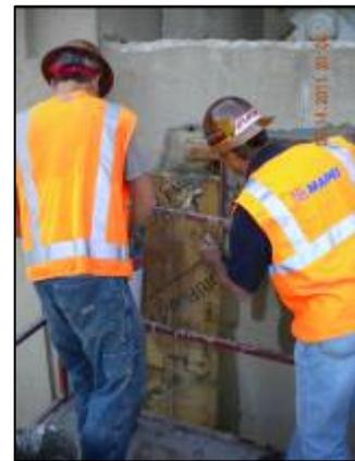
outer most reaches of the forms, they were lightly vibrated. In some areas, the mortar had to flow over 4 feet from the head box.
