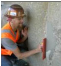
While the *Planitop* 15 was curing, the Gerber crew took care of smaller repairs using *Planitop X* – a non-sag, fast-setting, ‘sculptable’ repair mortar.
