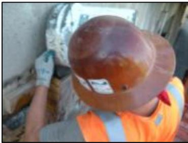
Due to the depth and volume of the voids, *Planitop* 15 was extended with 25 lbs. of washed pea gravel per 50-lb. sack and modified with *Mapecure SRA* shrinkage-reducing additive. The mixed mortar was then poured into the forms via head boxes strategically placed at the top of each of the forms. To ensure complete flow into voids as well as to the
