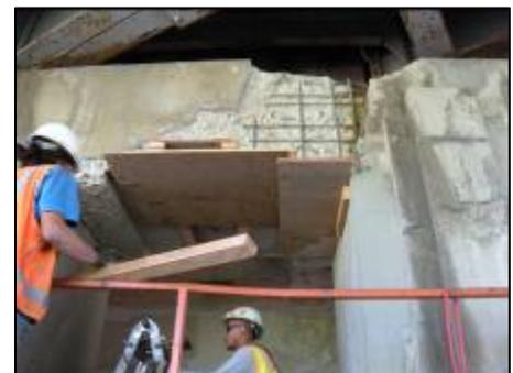
steel was either cleaned or replaced as needed, and forming was tightly fitted against the beams and columns to maintain the unique contours and shapes originally cast into the bridge.
