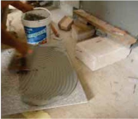
**TO THE LEFT.** Slabs of granite were covered around the edges of the ponds using KERAFLEX MAXI S1 and KERACOLOR FF.
