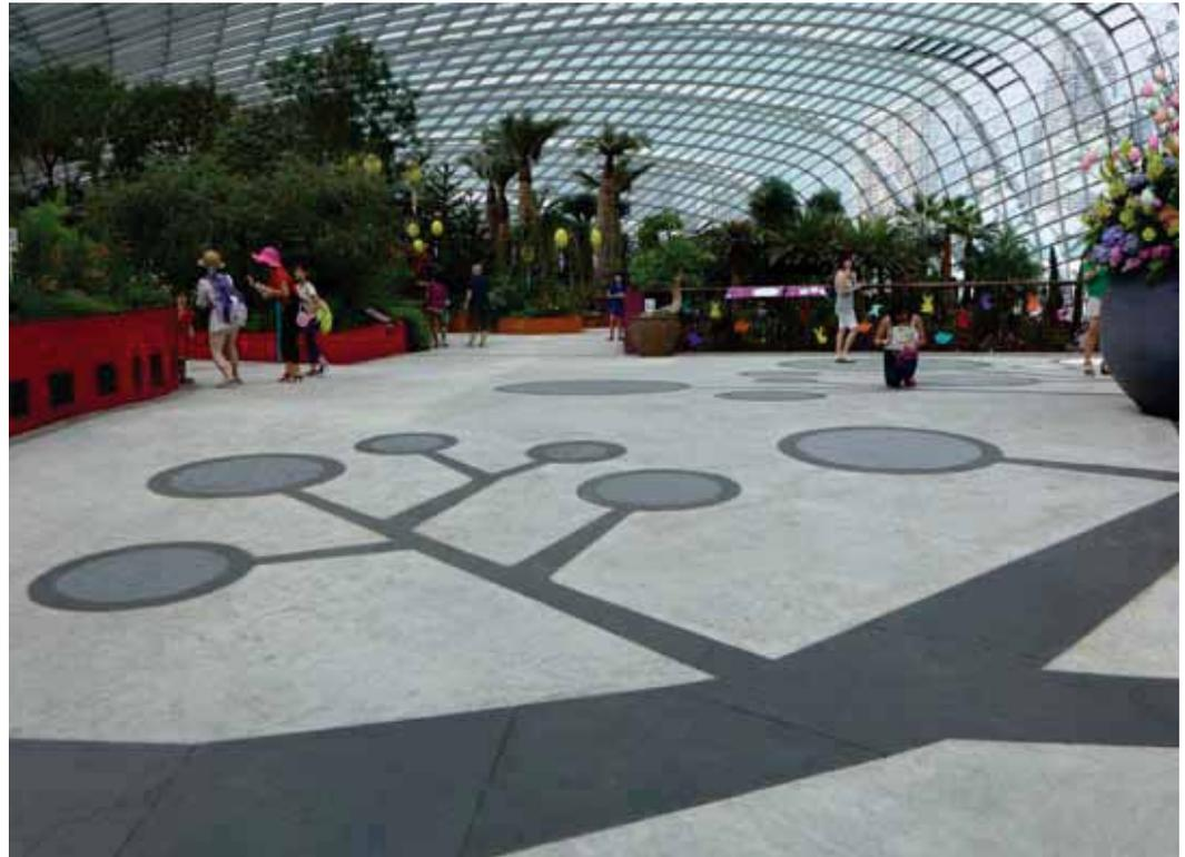
**PHOTO ABOVE.** The slabs of granite for the entrance of the Flower Dome were laid using KERAFLEX MAXI S1 and grouted with KERACOLOR SF.
