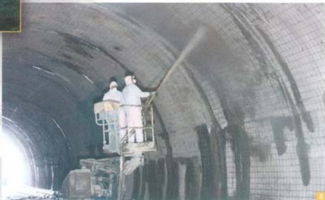
Photo 3. Technicians busy spraying on Mapegrout Gunite. You can clearly see the electrically welded steel mesh forming the frame for the plaster made from Mapegrout Gunite. The product was applied using a rotary pump directly supplied by bags of dry product hydrated when emerging from the hose.
