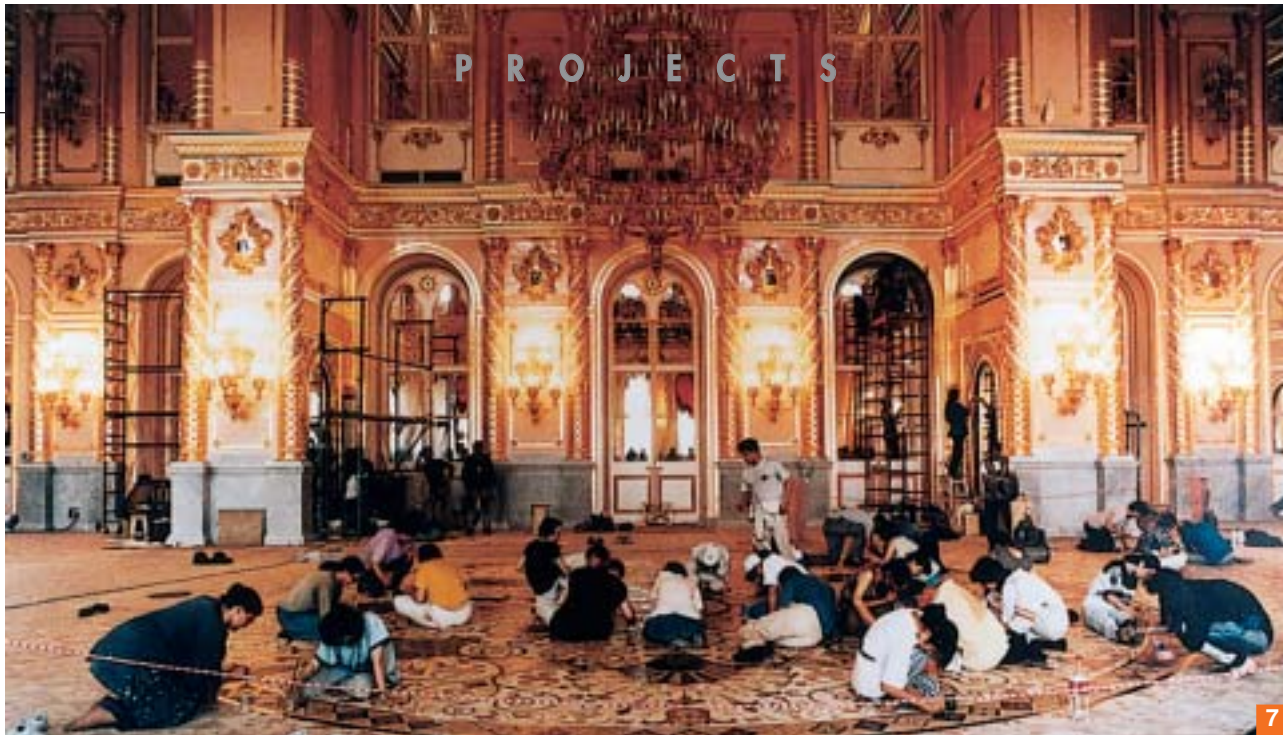
Photo 7. The restoration of the large central inlaid work in the Room of Saint Alexander.
