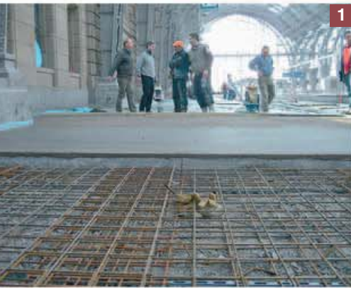
Photo 1. Preparing the concrete substrate reinforced with metal meshing.
