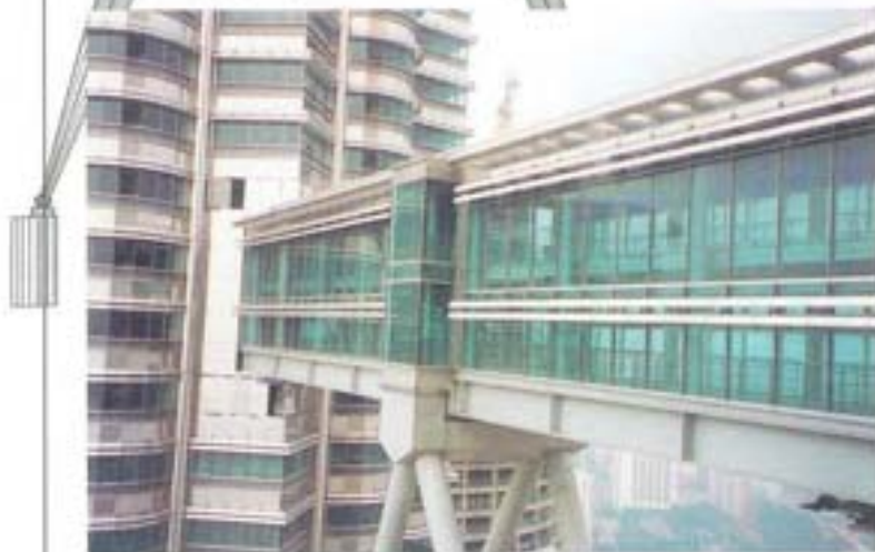
Perspective view and detail of the panoramic bridge suspended at a height of 171 m that joins together the towers at the level of the forty-first floor
