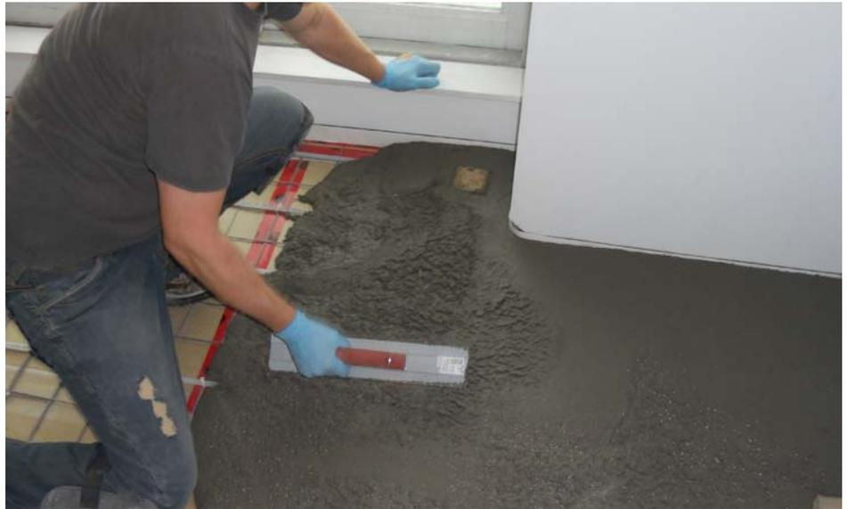
up into grids using high density foam. The foam strips were bolted to the slab and acted as screed rails for the mud bed. The mixing of the Topcem was done with a mortar mixer out on the small patio deck. (It was a challenge to dismantle the mixer and then re-assemble it out on the deck.) The mud bed installation was a two-day process.
