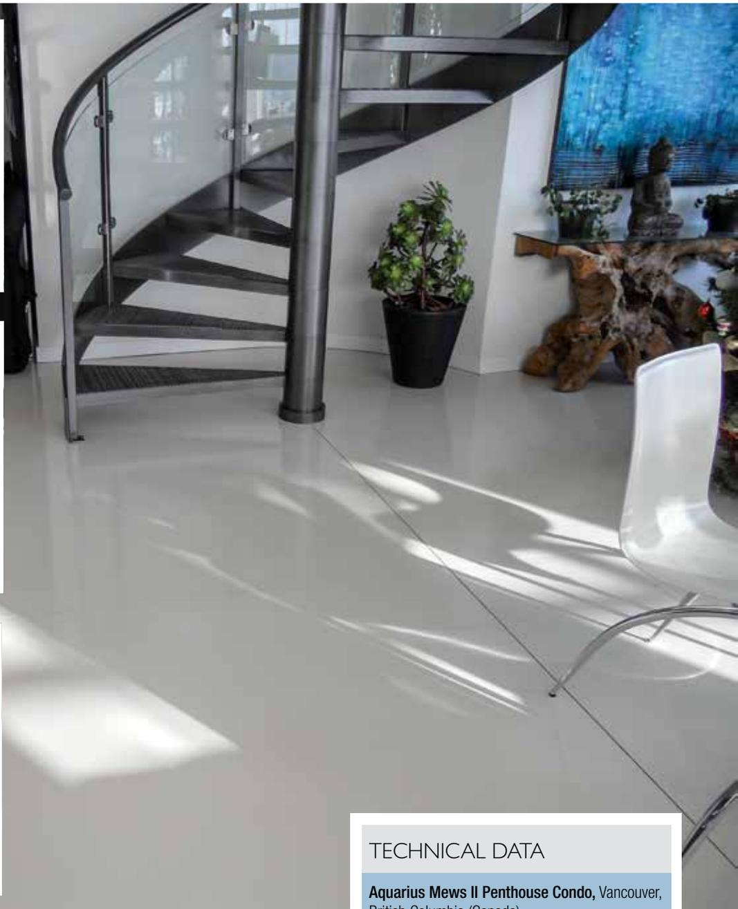
Next, the *Topcem Premix* mud bed was allowed to cure for two days before the overlay application. Workers applied *Primer E*™ with broadcast sand over the entire floor area of the condo unit, including the kitchen, hallways, bathrooms, closets and bedrooms. *Ultratop White* was then installed over the primer on the following day.
