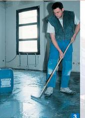
A fine-toothed trowel was used to apply the adhesive to the floor. This ensures the grooves are evenly distributed over the PVC surface after installation, forming a smooth film preventing any trowel lines from appearing on the coating.
