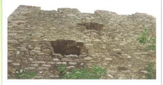
There were two stages of renovation; sealing the stones with MAPE-ANTIQUE MC, a mortar designed for historic buildings, followed by the consolidation, with injections of MAPE-ANTIQUE I, a binder also designed for historical building masonry.
