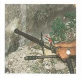
On the left, preparation of the MAPE-ANTIQUE I slurry bond coat directly in the special injection pump; executing the consolidating injections with MAPE-ANTIQUE I; detail of the hole after the injection. Below, the tower is ready for a new use
