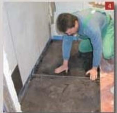
and floating screeds. Within only 4 days the screed was completely dry, after having hardened within 24 hours.
