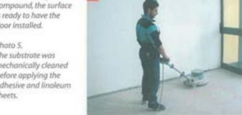
ultra-fast hardening self-levelling compound with low emission of volatile organic compounds (VOC). The photos show various stages in the process: the product is prepared for use by mixing it with water, before applying it to the substrate, 12 hours after applying the self-levelling compound, the surface is ready to have the floor installed.
