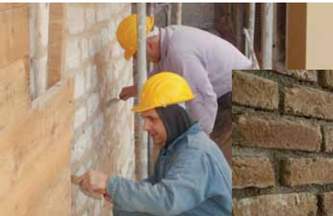
The original natural stone walls were consolidated with MAPE-ANTIQUE I-15 cement-free hydraulic binder.
