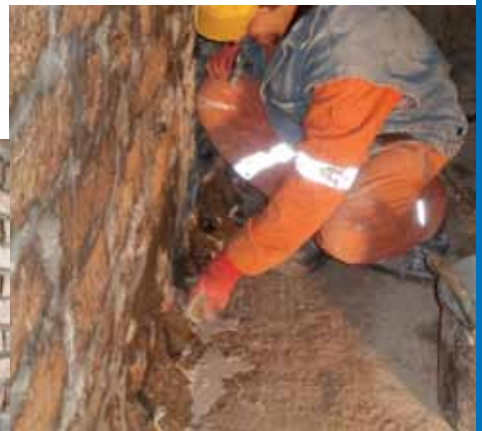
The original natural stone walls were consolidated with MAPE-ANTIQUE I-15 cement-free hydraulic binder.
