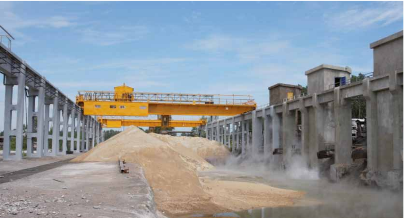
The sight of the slag drop zone construction after renovation.
