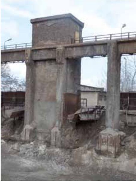
Zone I. Concrete degradation in the slaking slag construction installation.
