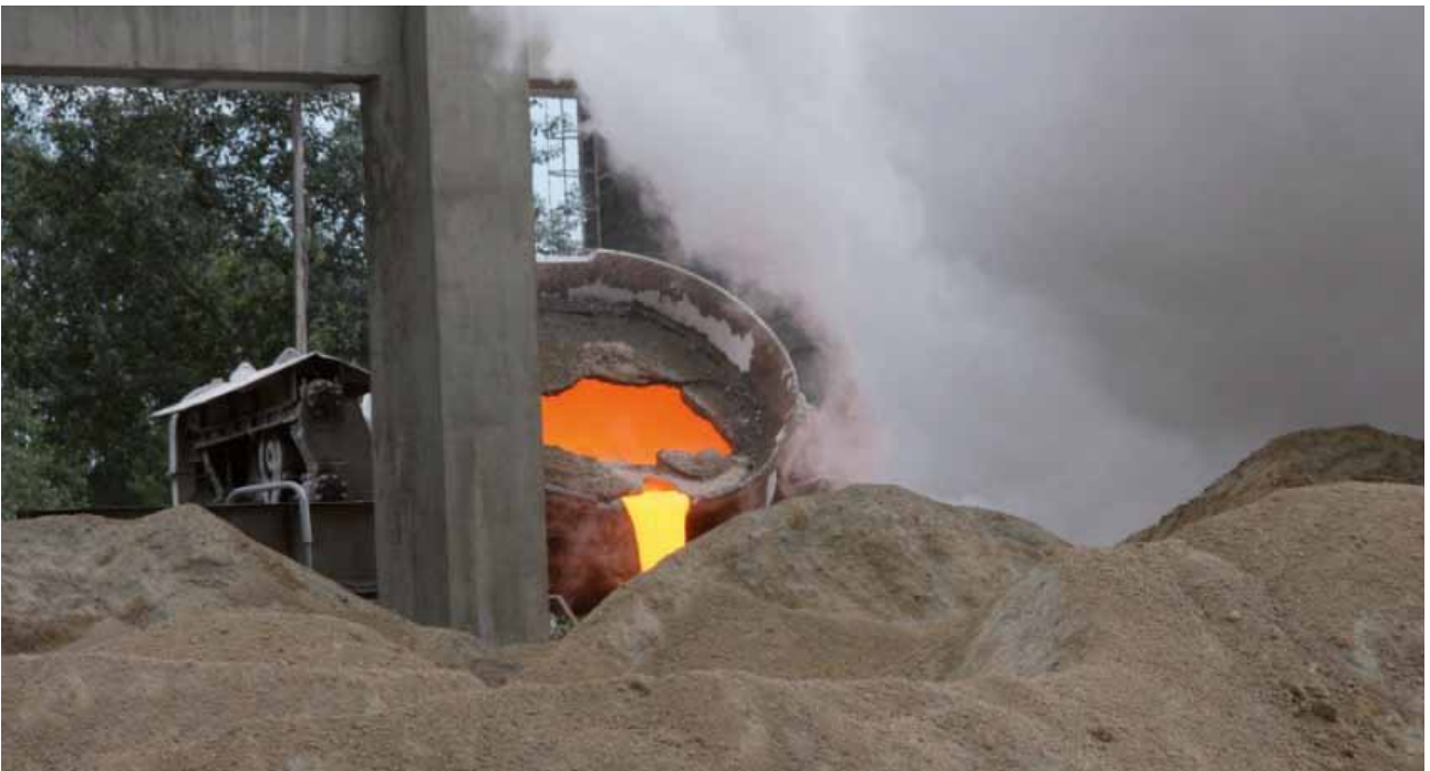
The detail of the slag drop zone construction after renovation.
