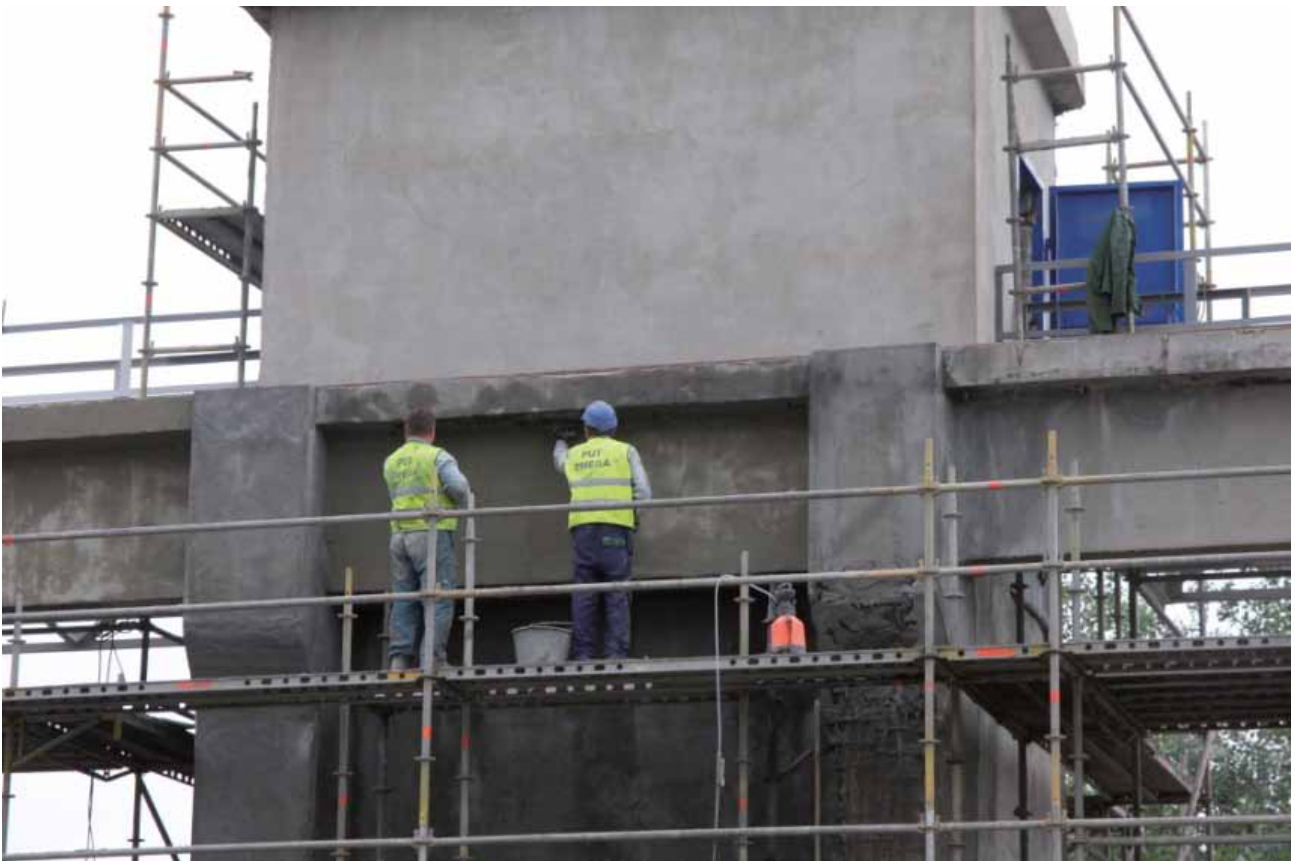
Repair works in the slag drop zone construction.
