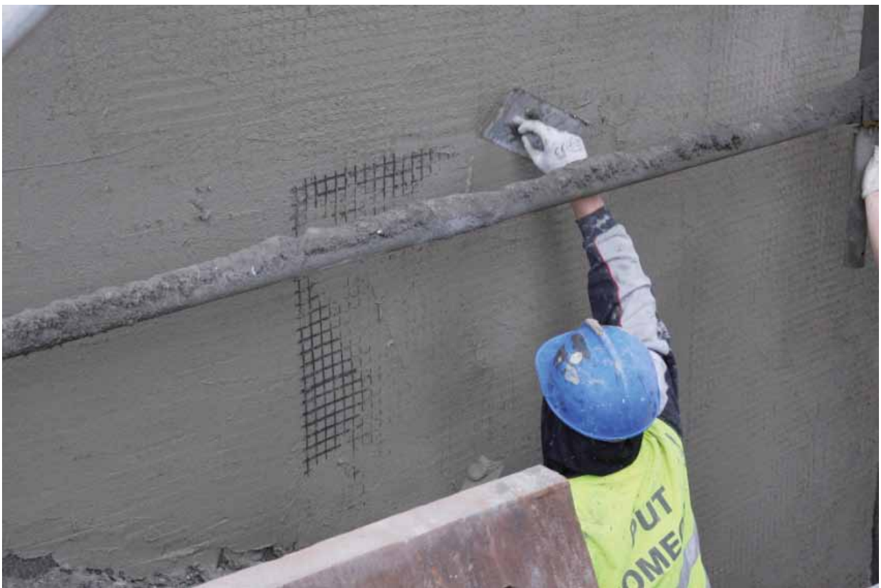
Immerging the alkali-resistant mesh in the cementitious-polymer mortar.
