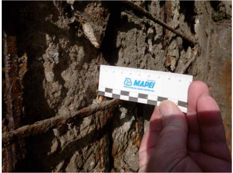
Zone I. Concrete degradation in the slaking slag construction installation.
