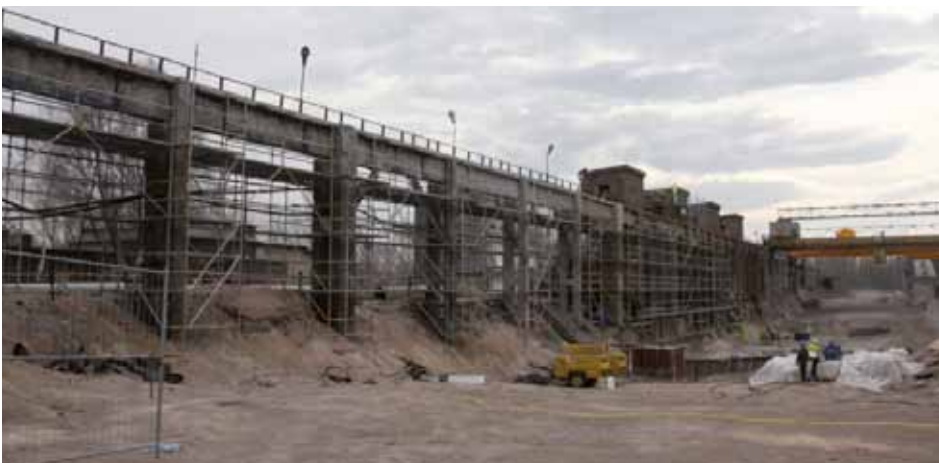
The concrete structure in the slag drop zone.
