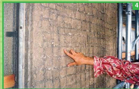
Photo 4. Complete detachment of the installation mortar and, therefore, of the glass covering leaving the levelling concrete visible.
