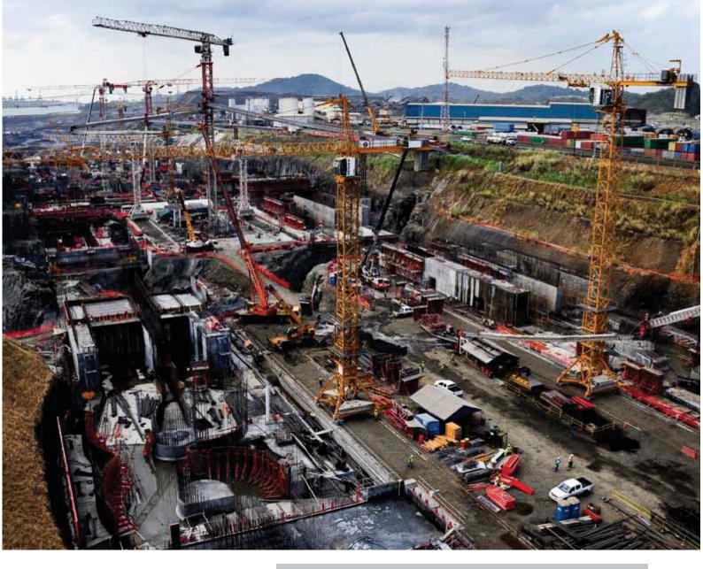
**Above.** Mapei admixtures were selected to make the mass concrete structures and for the marine concrete to be used to make the external sides and internal sides the concrete locks, respectively.
