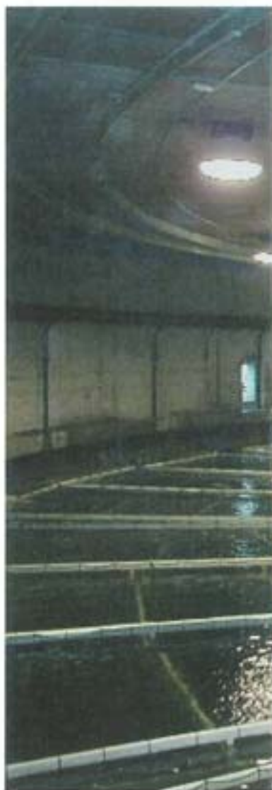
6. Fry tank covered with MAPELASTIC (before final cleaning)
