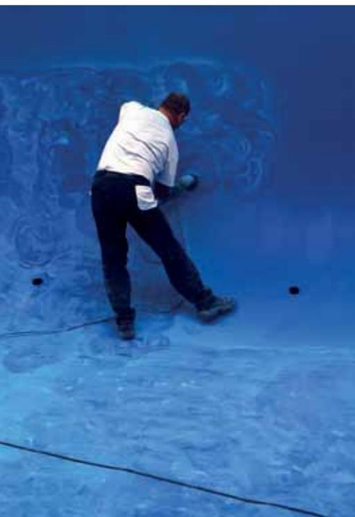
of PRIMER SN, two-component epoxy primer, fillerized with QUARTZ 0.25 to act as adhesion primer.
