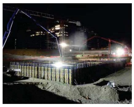
3K viscosity modifying admixture, to form a C32/40 LH XC2-XC4 SCC concrete with high self-compacting properties and controlled development of heat hydration.
