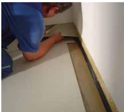
**Above.** ULTRABOND ECO V4 SP was used to install the Nora rubber floorings on the stairs in the east wing.
