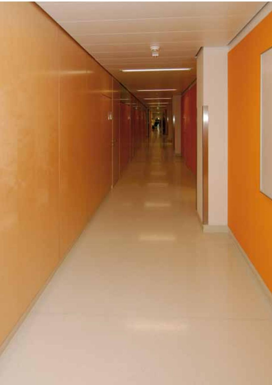
**Below.** The Nora synthetic rubber floorings in the corridors in the east wing were installed with ULTRABOND ECO V4 SP after preparing the substrates with PRIMER MF, ULTRAPLAN MAXI and ULTRAPLAN.
