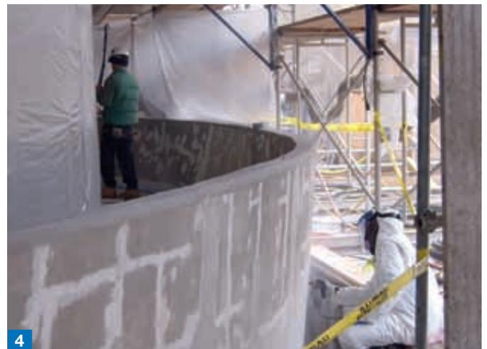
developed into expansion joints) and those caused by shrinkage of the concrete. It was obvious that the different types of cracks had to be treated using different operating methods. More generally speaking, Mapei was asked to deal with the building's structural problems.
