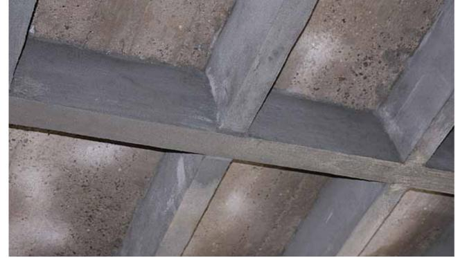
Fot. 1. Repair mortar PLANITOP 430 on concrete beams
