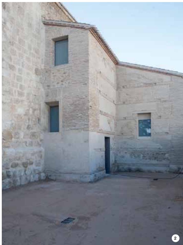
PHOTO 1. The external masonry walls at the start of the intervention.
