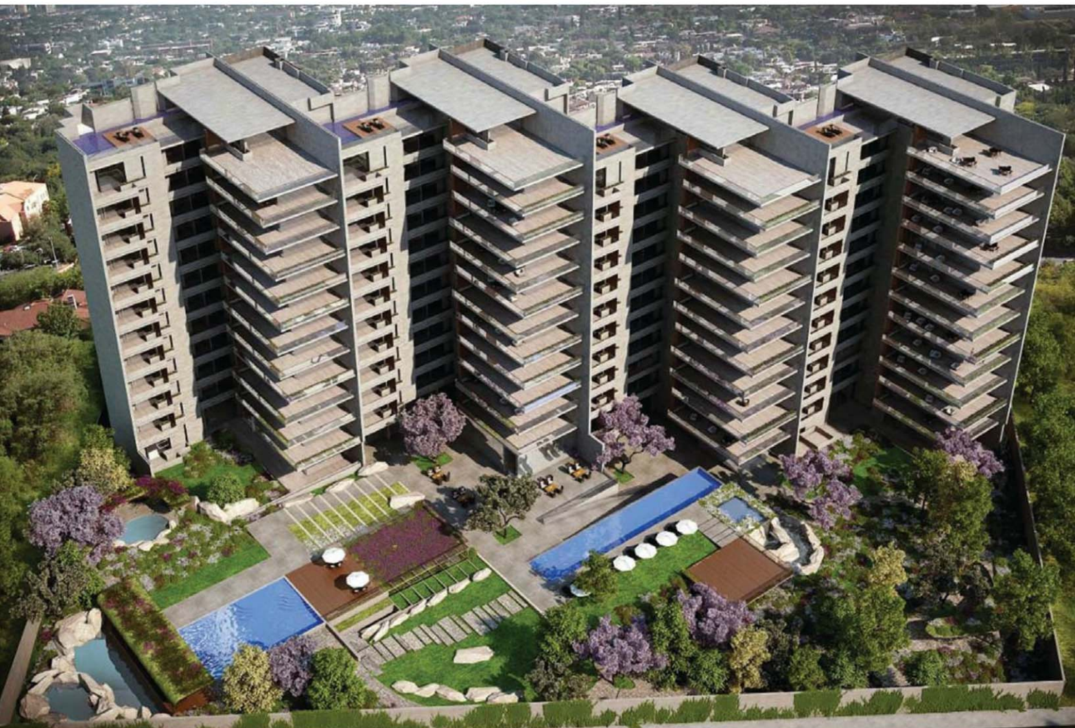
The El Alear Condominium complex in San Pedro Garza García, Monterrey, Nuevo León, Mexico, which were designed by Dr. Esteban Astudillo and architect Agustín Landa Ruiloba, comprises four connected buildings that house a total of 46 exclusive luxury condominiums, with a separate lobby for each of the buildings.
