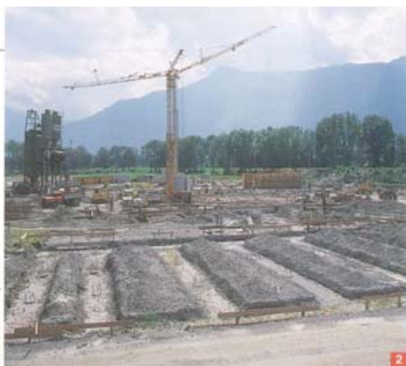
Photo 1. The inauguration of the new CMC. Photo 2. The first works phases. Photo 3. A view of the almost finished centre.
